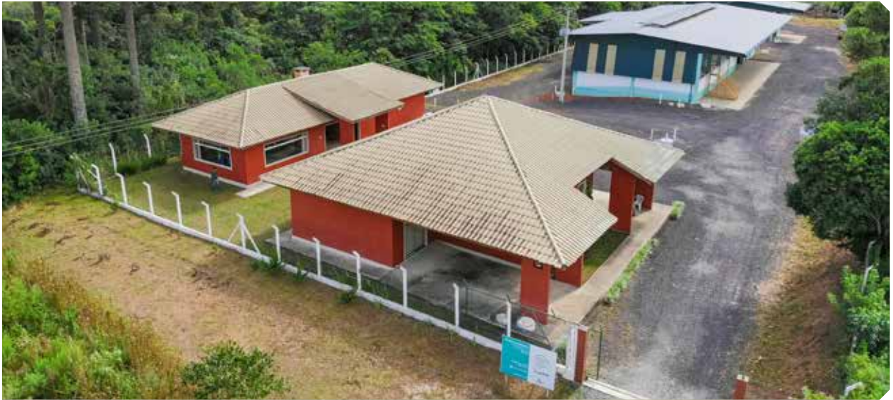
Receiving station of the Campo Limpo System in Contenda (PR), managed by inpEV.
